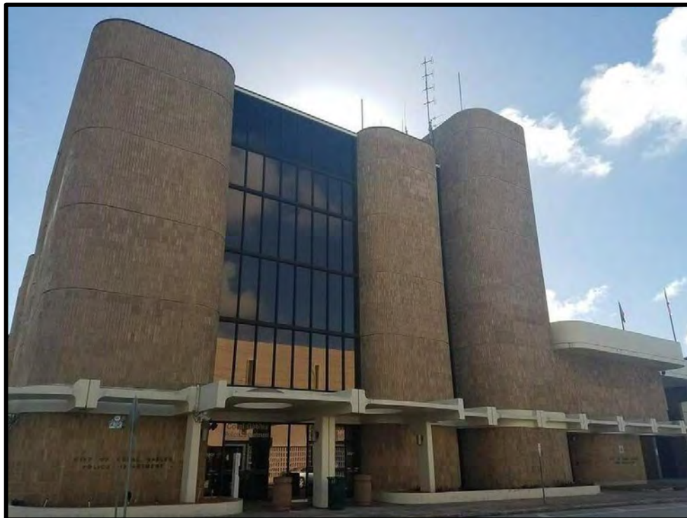
Existing Public Safety Building
