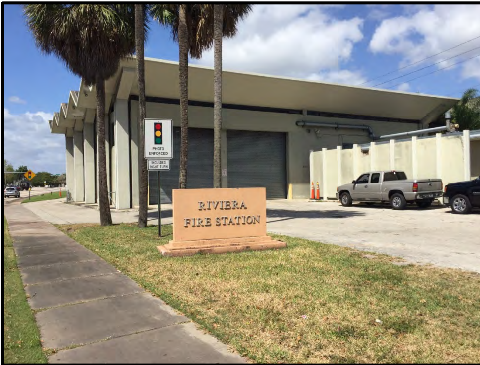
Current State of Fire Station 2
