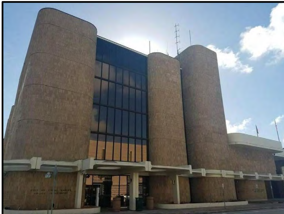
Existing Public Safety Building
