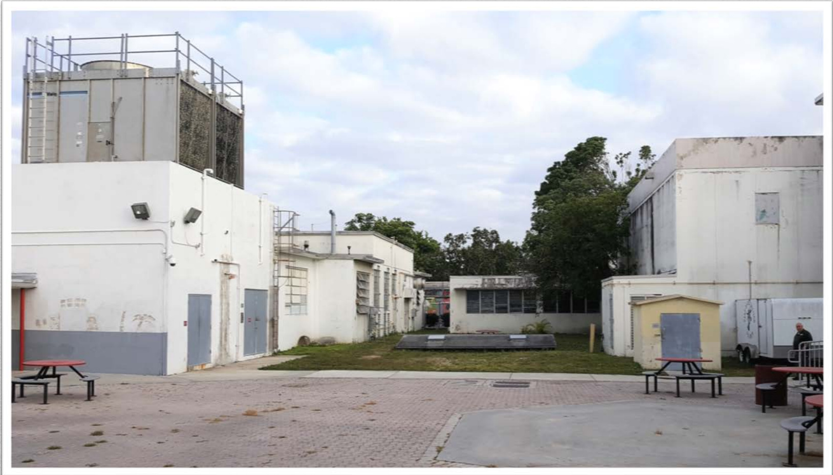
Existing – Chiller Plant
