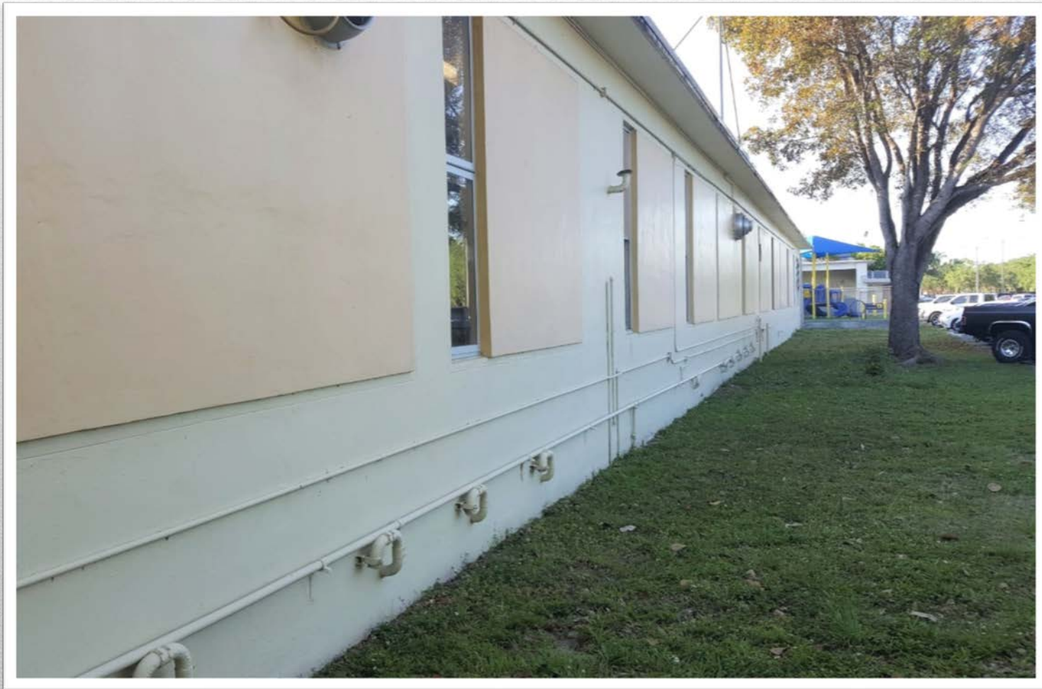
New windows and removal of plumbing lines
