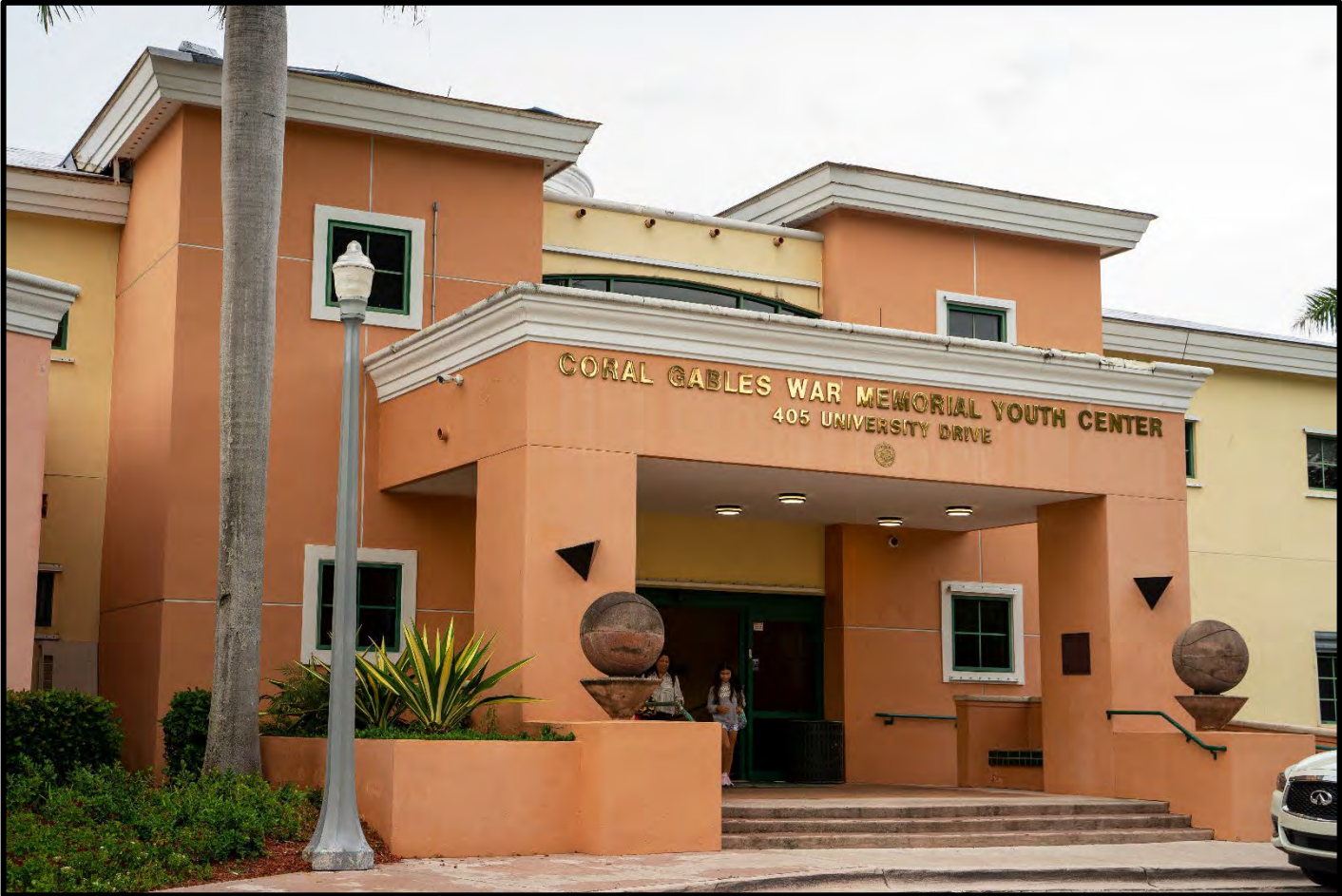
Youth Center Impact Glass Installation
