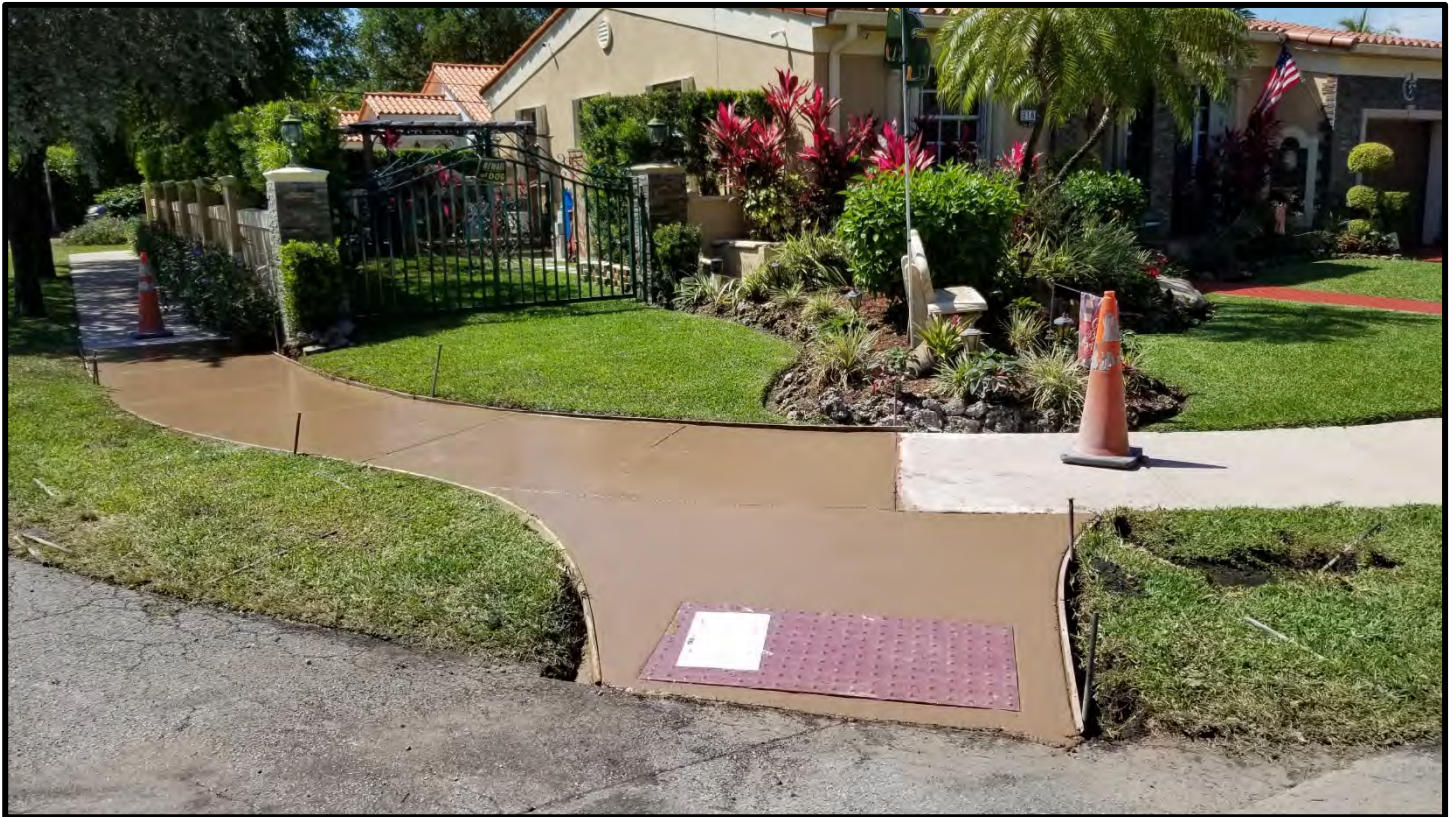
New Sidewalk Extension
